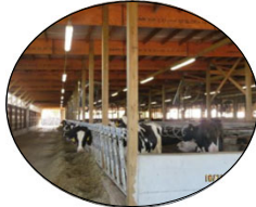
LED lights throughout facility
